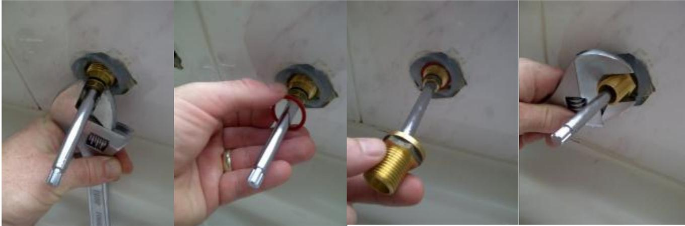
1. Screw in the ceramic cartridge by hand until it reaches the tap seat. Then gently tighten with a spanner at about the same strength you would use to turn off a tap. Place the fibre washer over and then tighten on the lock nut firmly with a spanner.
