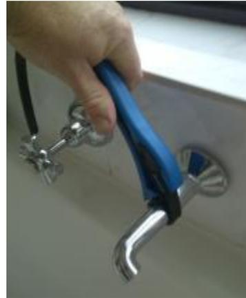
2. Remove the old spout. A rubber strap wrench is ideal for undoing tight spouts. Another way is to insert a screw driver into the outlet and use it as leverage to undo it.
