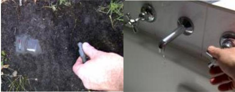
1. Turn off the water at your meter and drain your system by opening the lowest hot and cold outlet in your house. Usually the bath taps.
