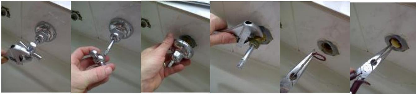
3. Undo the old handle, flange, spindle and make sure you remove the fibre body washer and jumper valve. The old jumper valve may have swollen so the pointed nose pliers will make removal easier.
