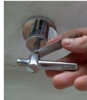
2. Turn off your taps if they are running. Select the angle at which you want the lever to be when switched off. Now simply tighten the discreet locking nut with the anti vandal spanner.
