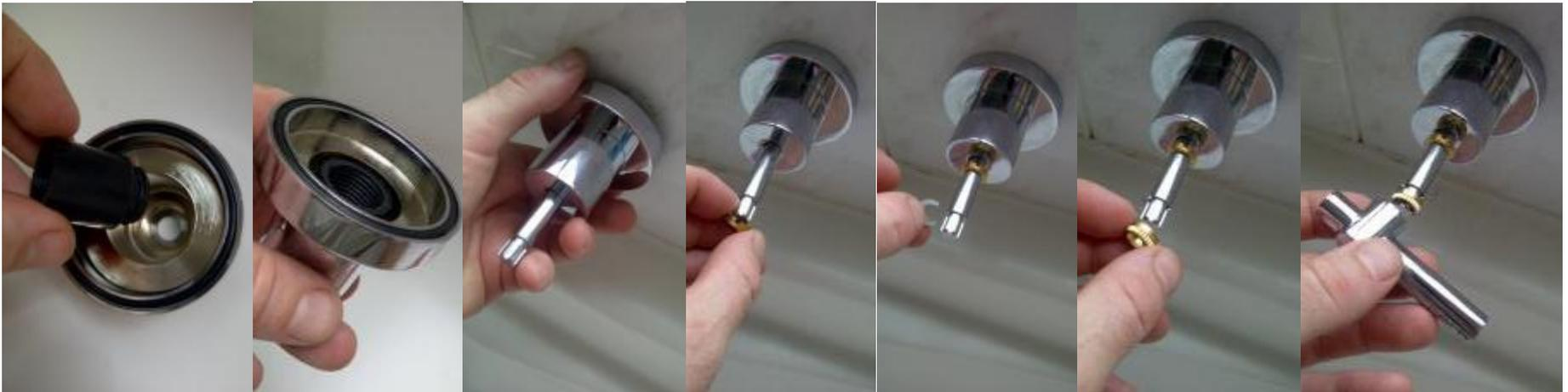
2. Screw the pvc thread extender into the tap flange and re-install. Push on the discreet locking nut, circlip, handle adaptor and then handle.
